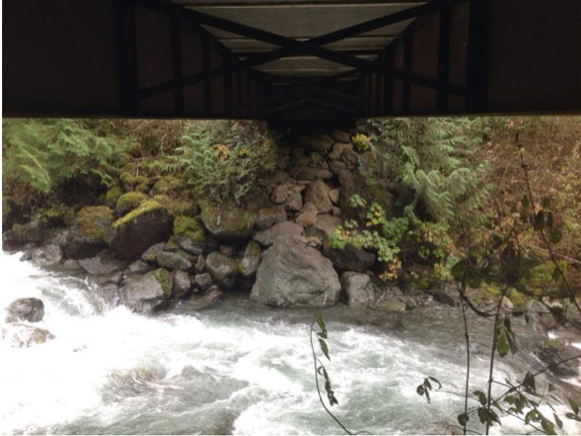
Left Bank Abutment when facing downstream
