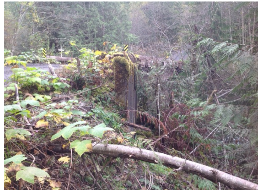
precast wingwall downstream right bank
