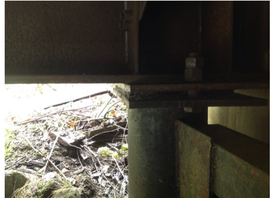
left bank bearing pads - typical both sides
