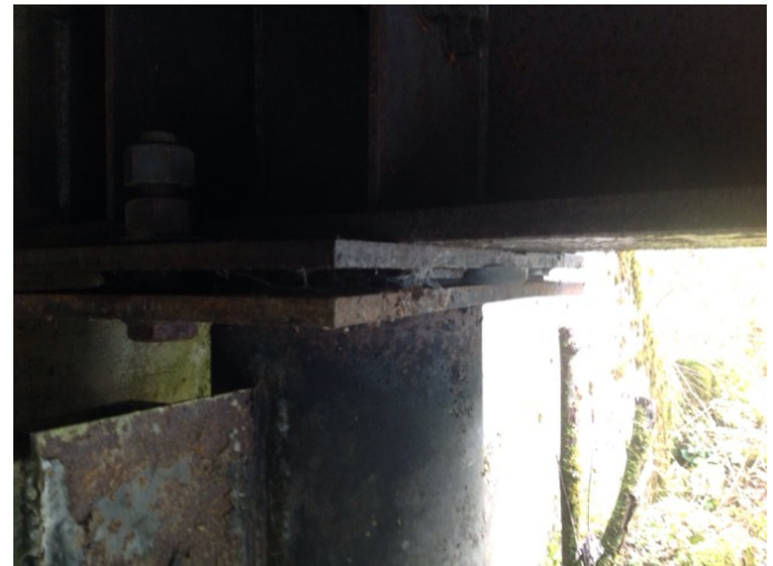
right bank bearing pads - typical both sides
